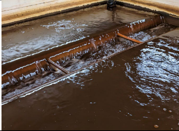
Figure 1 – Water leaving the bead chamber after air-scour and flushing.
